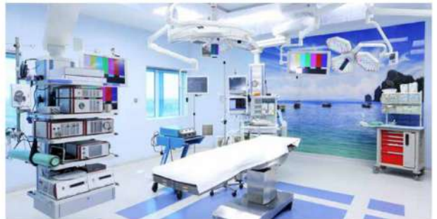
Aims Hospital, Nagar
